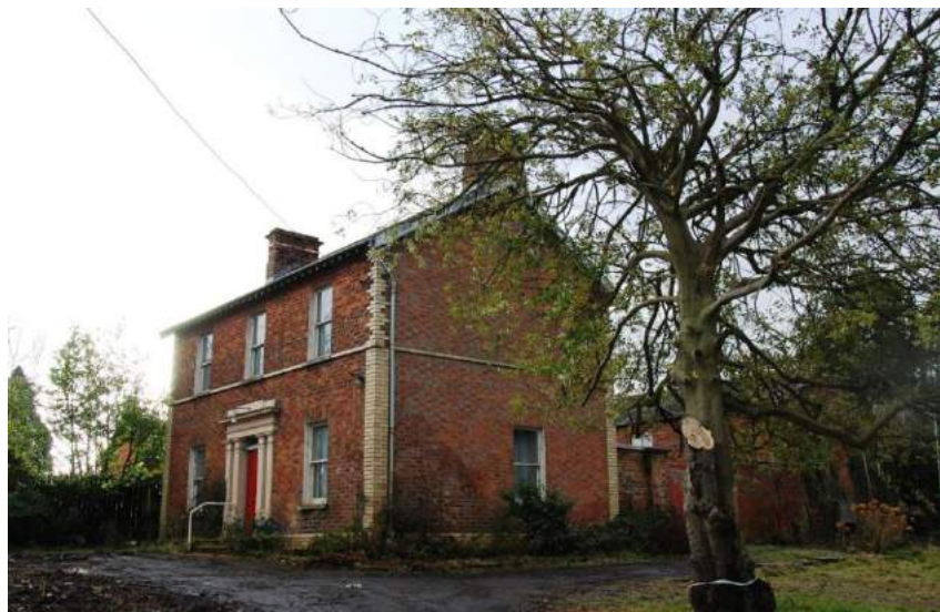
Above: Navigation House, 134 Hillsborough Road, Lisburn © DOE
