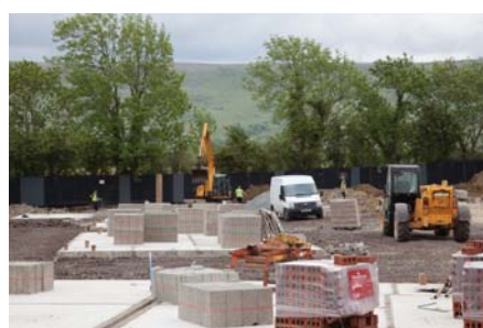
Social housing at Hass Road, Dungiven (Phase 1 completed and Phase 2 under construction)
