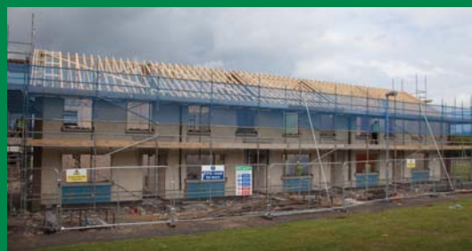
Extensive refurbishment of social housing at Mossvale Park, Ballysally
