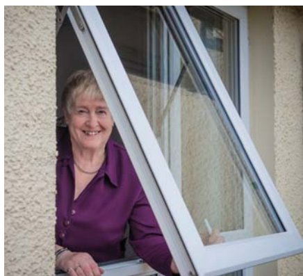
New double glazing installed in Housing Executive homes in Ballymoney in the past year
