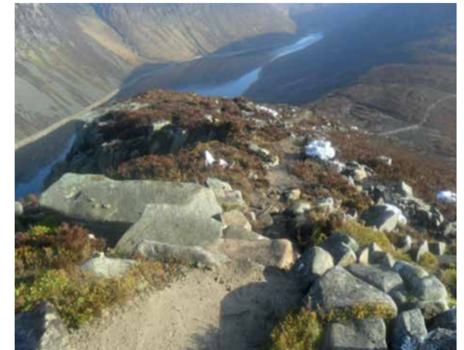
Upland Path Works on Binnian Mountain
