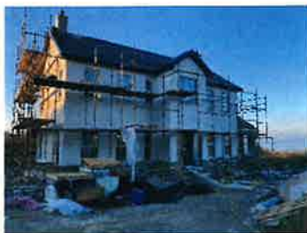
Image 1 new build complete
