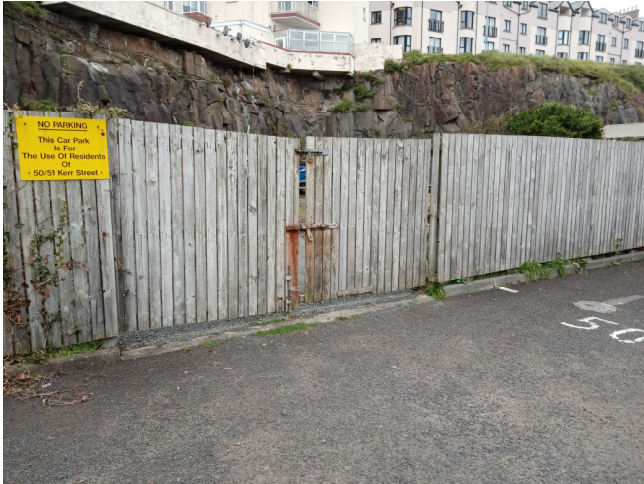
Figure 1 – Site Boundary & Gates
