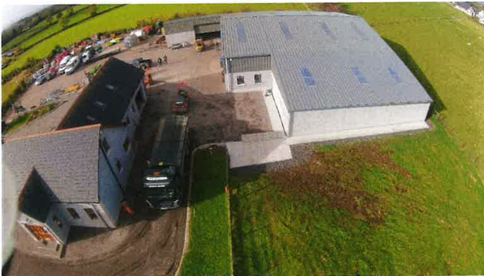
Photograph 5 – Drone photograph taken August 2015 of Building 3 completed.
