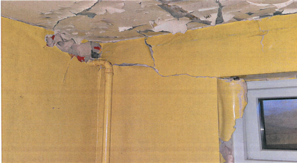
Photo 6 – Internal Cracking
