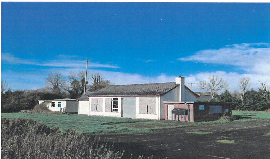
Photo 1 – External view showing main hall and ancillary accommodation
