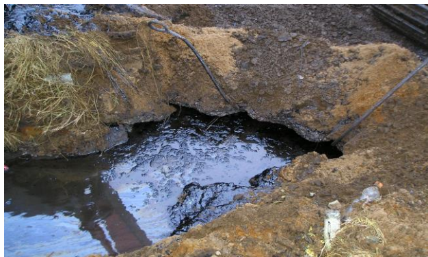
Photo – Depicting Coal Tar* from Former Gas Works Site – Seepage from Underground. * Coal Tar is a Source of Contamination (Cocktail of Harmful Carcinogenic Substances)
