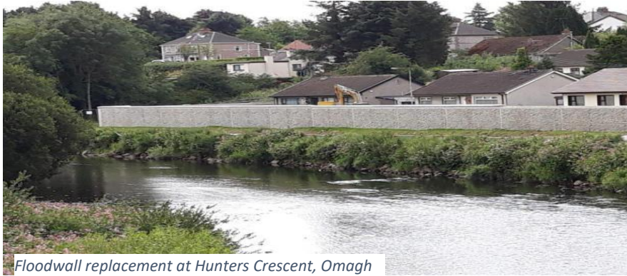
Floodwall replacement at Hunters Crescent, Omagh
