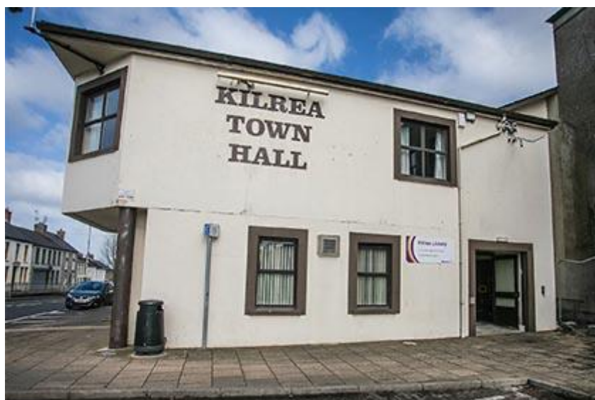
Figure 4: Kilrea Town Hall
