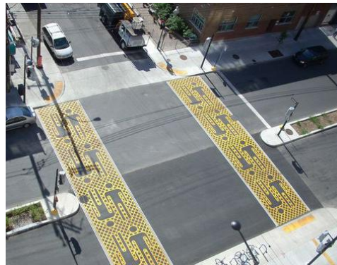
Improved demarcation of street crossings
