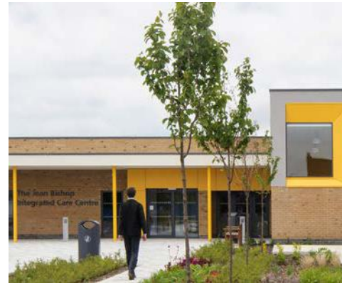
Integrated Care Centre
