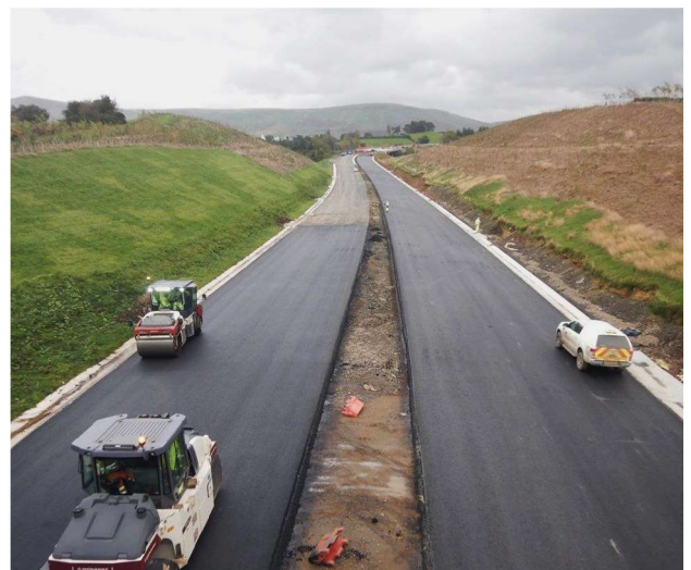
Construction of dual carriageway at Magheramore.
