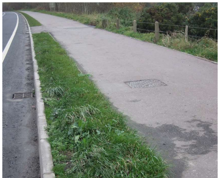
Foreglen Road, Ovil, Dungiven – Completed scheme.
