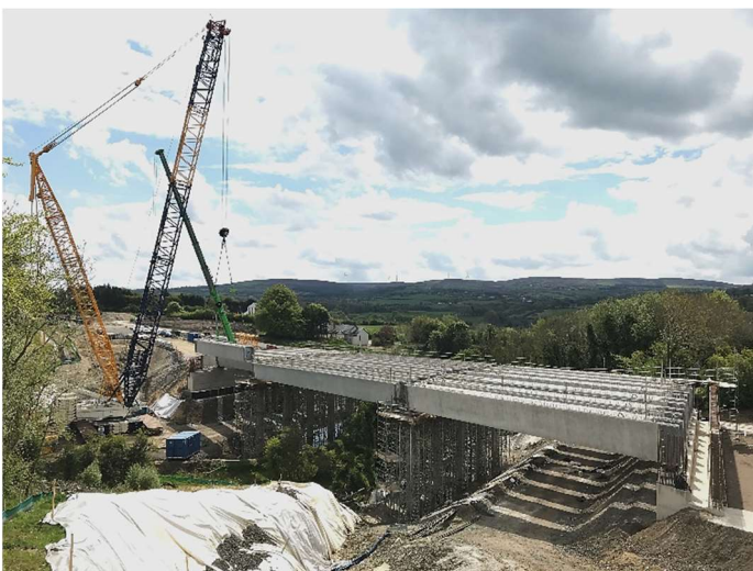
Beams being lifted in place for the Liberty Glen bridge.
