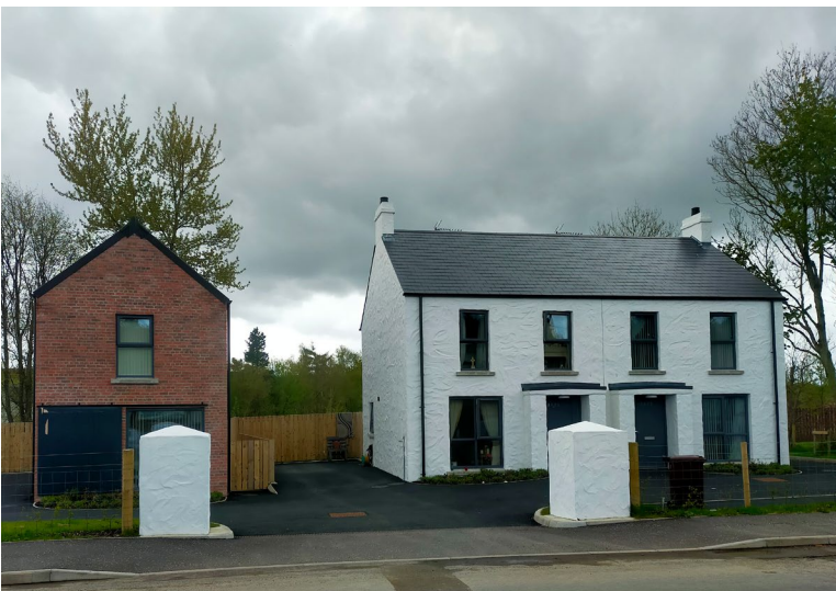
Foreglen, (Rural scheme) site adjacent to 299 Foreglen Road, Rural Housing
