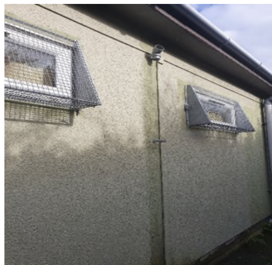
Figure 14 – Missing Downspout
