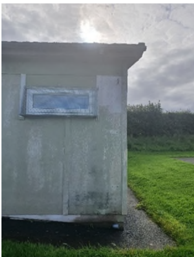
Figure 13 – Missing Downspout
