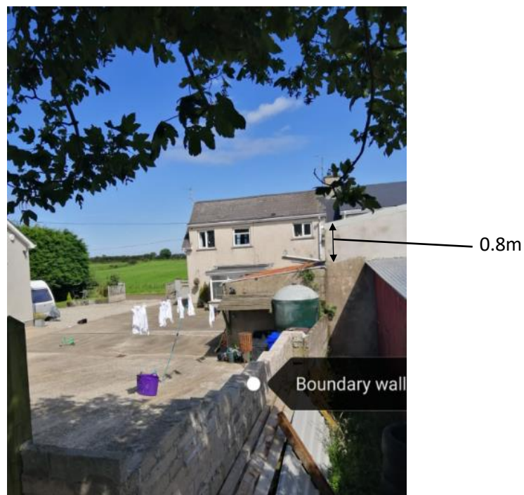
Photo 8: View of garage from rear
