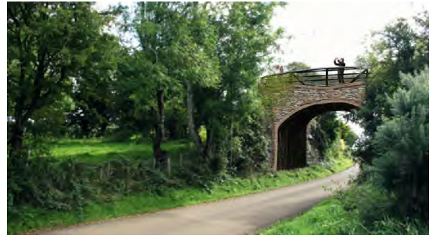
New Bridge on Hillside Road
